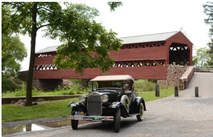
The Sachs Covered Bridge, Freedom PA;
